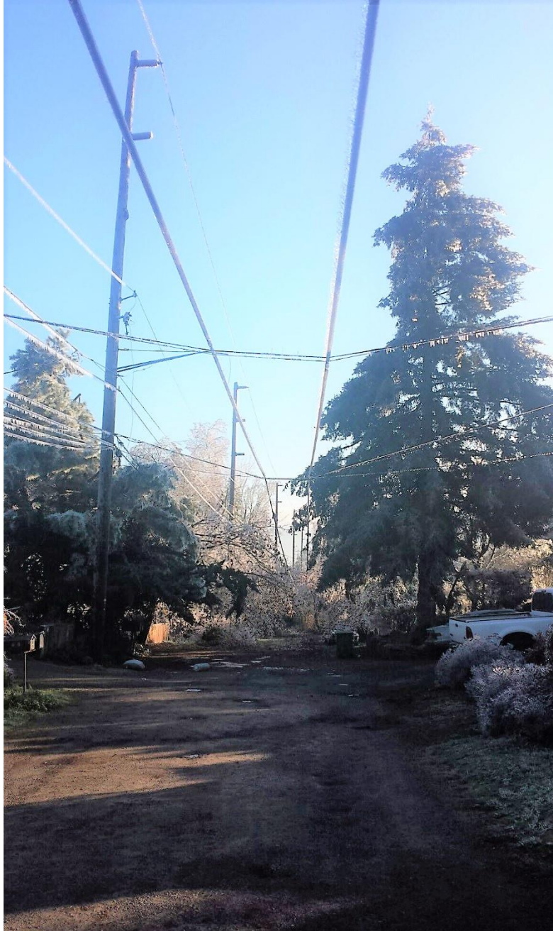
Figure 2: Downed line supported by communications lines.
